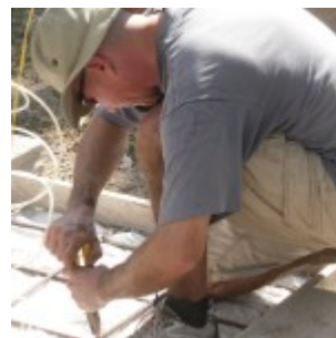
Nathan wiring the rebar
