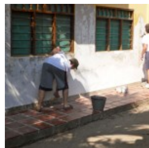
Cleaning the wall
