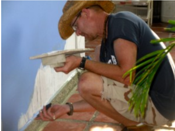
Jay plastering the wall
