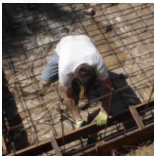
Nate working on the forms
