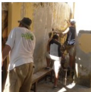
Scraping and cleaning
