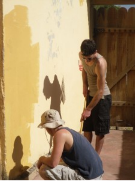
Jesse and Sam working on the wall
