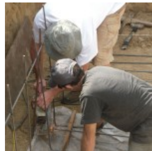
Vic & mark cut rebar
