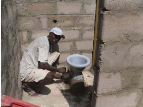
Luis working the finish of the concrete
