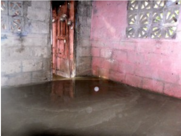
The finished floor
