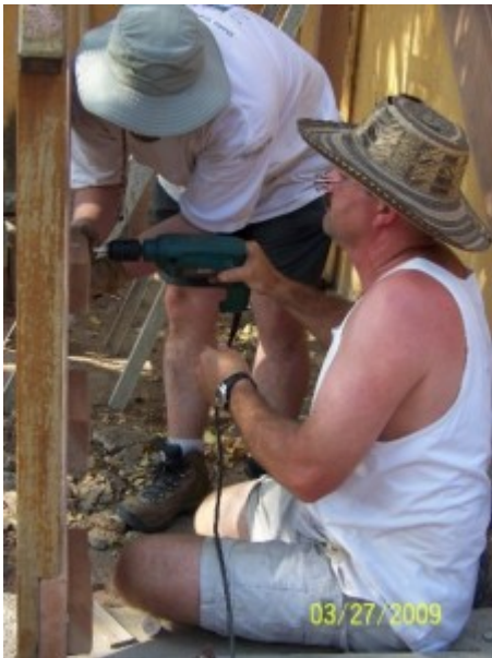
Thom and Geoff building stairs
